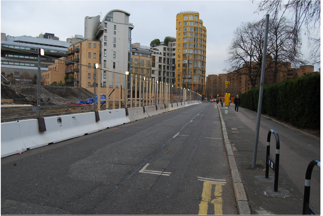
Holland Street – Neo Bankside site on the left (west), Tate on the right (east), and the new Thameslink Blackfriars station to the north
